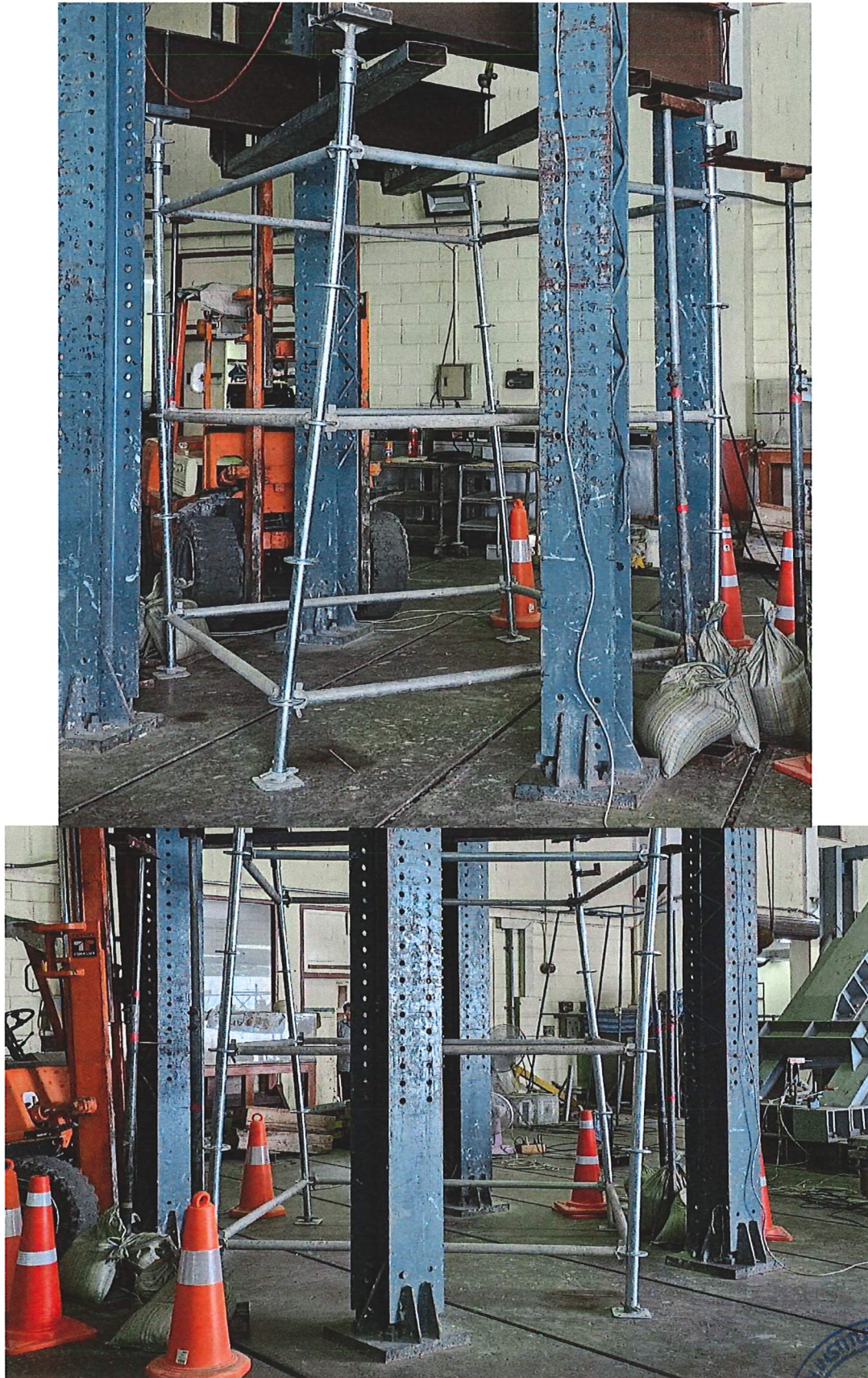
Figure 4 Specimen condition at maximum load
